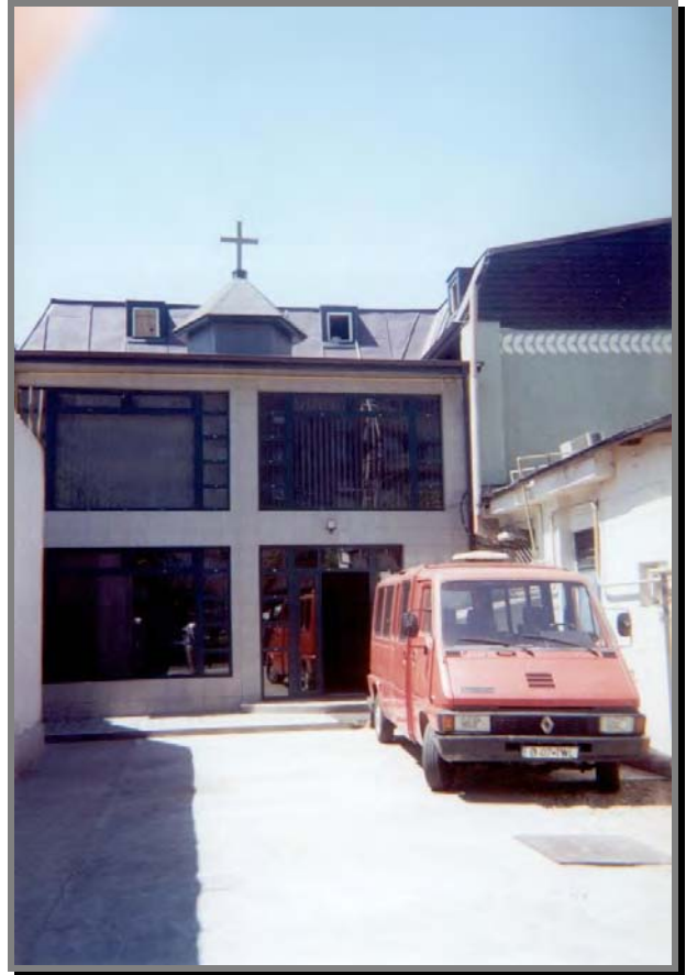
Reformed Theological Institute facility is three-storey high, with the third floor children ministries, Hong's office, second - with classrooms, admin office, first - with kitchen, dining room, and unused offices.
